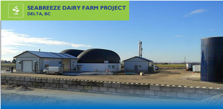
Waste from Lactalis' Delta yogurt plant is converted to energy through the biogas plant at Seabreeze Farm, powering 500 homes in the area.
